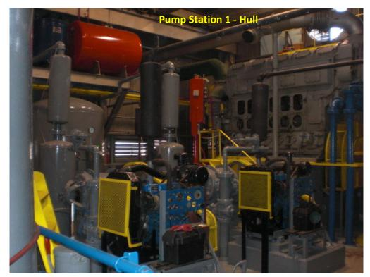
accumulated over that 3 1/2 year period, the equipment suffered a lot of wear and tear. Both pumps at Pump Station #1 repaired were along with one of the gearboxes. Two gearboxes and two pumps at Pump Station **3A** underwent which repairs, were finished this year. Once repairs
