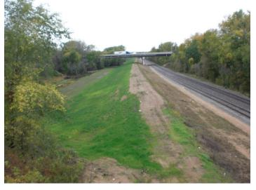
extremely dry conditions this year was re-sloped and seeded to provide protective sod cover on the river side. This image might best describe 2012: REPAIR AND MAINTENANCE.
