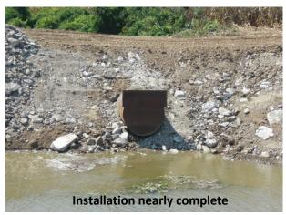
welded. The flapgate was adapted in the field
