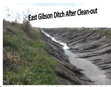
Ditches is limiting the amount of siltation that enters the ditch. We have found that the use of drainage tubes to direct the water from field drains to ditches rather than having the water run directly into the ditch dramatically limits the amount of silt
