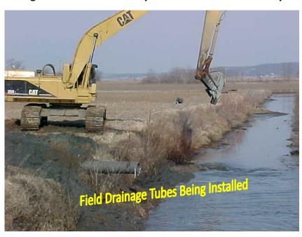
deposited into the The image ditches. on the left shows the installation of field drainage tubes into areas that formerly drained directly into the ditch. Please note in the background the deposit of silt into the ditch from fields draining directly into the ditch.
