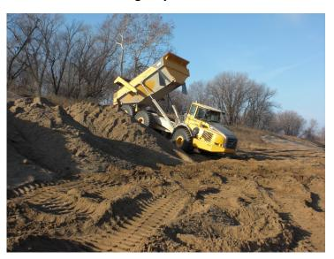
dredge project began so barge traffic could resume. Approximately 17,000 cubic yards of sand was taken from the channel and stockpiled on the land side slope of the river levee in an area locally known as the "Hackler Farm". It was then loaded on the quarry trucks and hauled to various nearby areas to address slope Then the Corps hydraulic dredge "Goetz" was moved into the area to begin a more extensive channel
