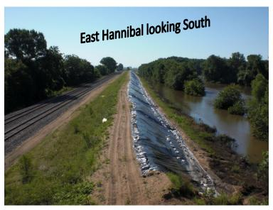
June 23 the decision was made to install plastic with sandbag anchors along a 1.1 mile stretch of levee in the East Hannibal area where seepage is particularly troublesome.
