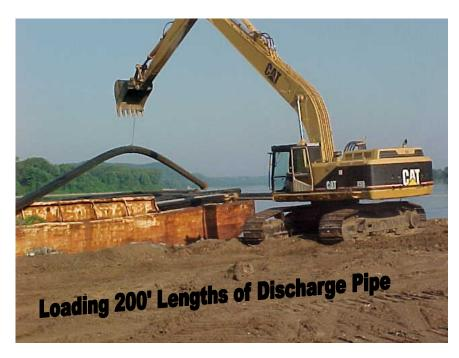
At the completion of Reach II, efforts were immediately initiated to move the entire dredging operation through Lock & Dam 22 upstream more than 16 miles to the north end of Reach I. By entire operation, we mean nearly 8,000' of discharge pipe, dredge, booster pump, work barge and workboat dock. The Sny enlisted the services of Caldwell
