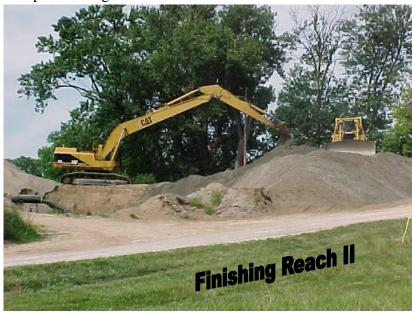
2007, dredging operations for strengthening the main stem river levee in Reach II was completed. Shown on the left is the D6R and 350L closing the final section of levee south of the Cincinnati Landing ramp. Dredging work began in Reach II at the insistence of the U.S. Army Corps of Engineers. As a requirement to secure
