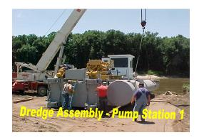
Sand hydraulically dredged from the river would be moved through 14" polyethylene discharge pipe to the landside slope of the levee. The 6,000' of pipe, delivered in 50' sections, were fused together in 200' sections with a \$29,000.00 fusion machine
