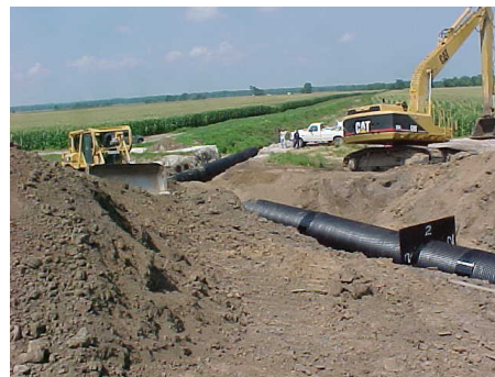
District Staff Installing New Outlet In Austin Creek Basin
