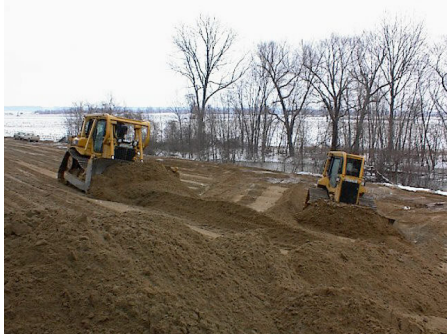
Cat D6R and D5M Shaping River Levee
