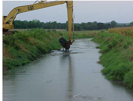
Cat 350L Trackhoe Cleaning Collins Pond Ditch
