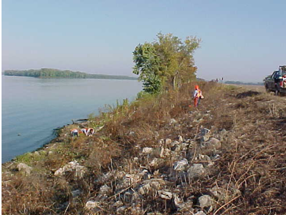
Pittsfield Work Camp Crew Clearing Riprap – Reach III
