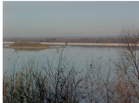
3.5 mile river levee riprap repair north of Lock & Dam 24 in Reach III as seen from the Missouri shore.
